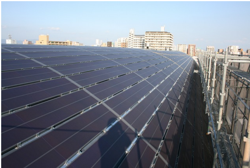
<Image of all-in-one panel solar cell attached on long folded-plate/undulate slate roof material>
